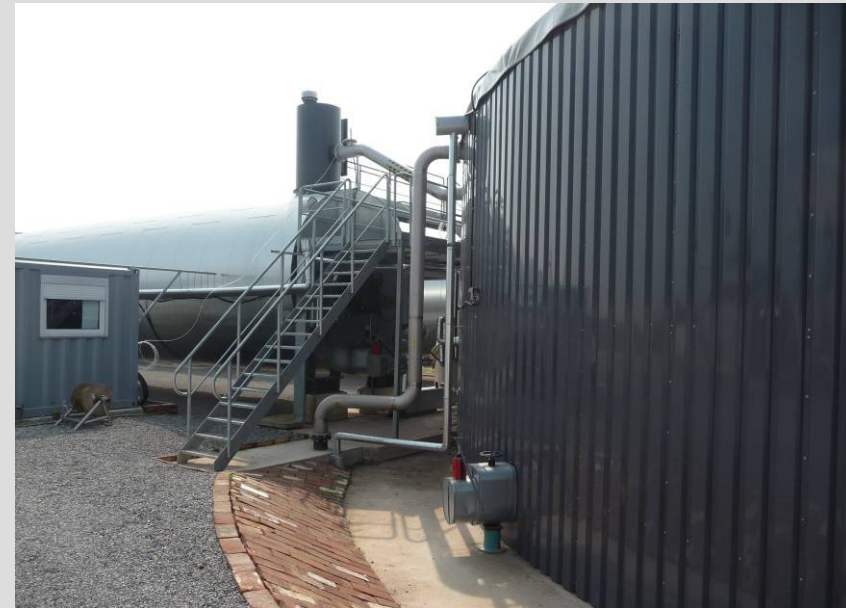
Inspection walkway for gas dome
