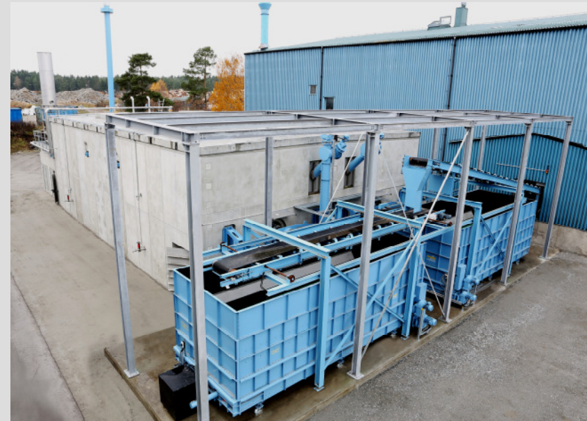
Double rectangular digester with sliding floor
