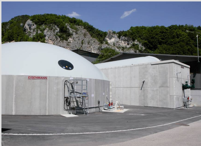
Main digester and final storage tank
