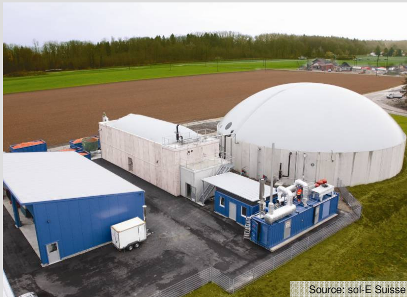
Aerial view of entire plant
