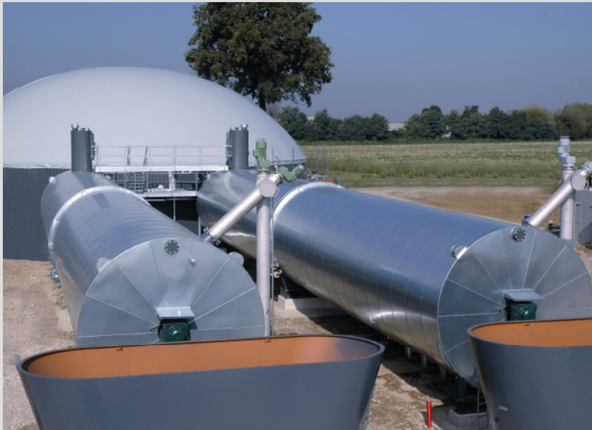
Main digester with solids dosing and post-digester
